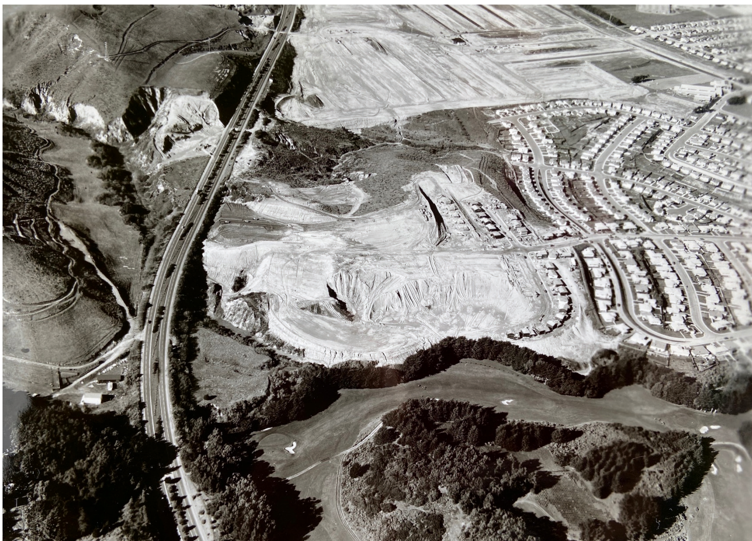
Massive grading for a large subdivision in the mid-1950s, likely in the San Mateo or Pacifica area, showing the clearing and filling of vegetated valleys and other areas. Courtesy Dave Holbrook.
