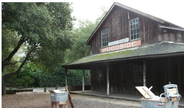
Woodside Store, constructed 1854.
