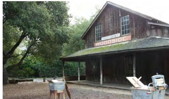
Woodside Store, constructed 1854.
