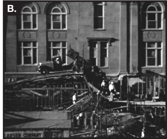
Building an addition in front.
