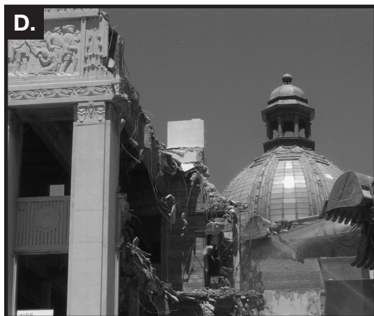
Tearing down the front addition.
