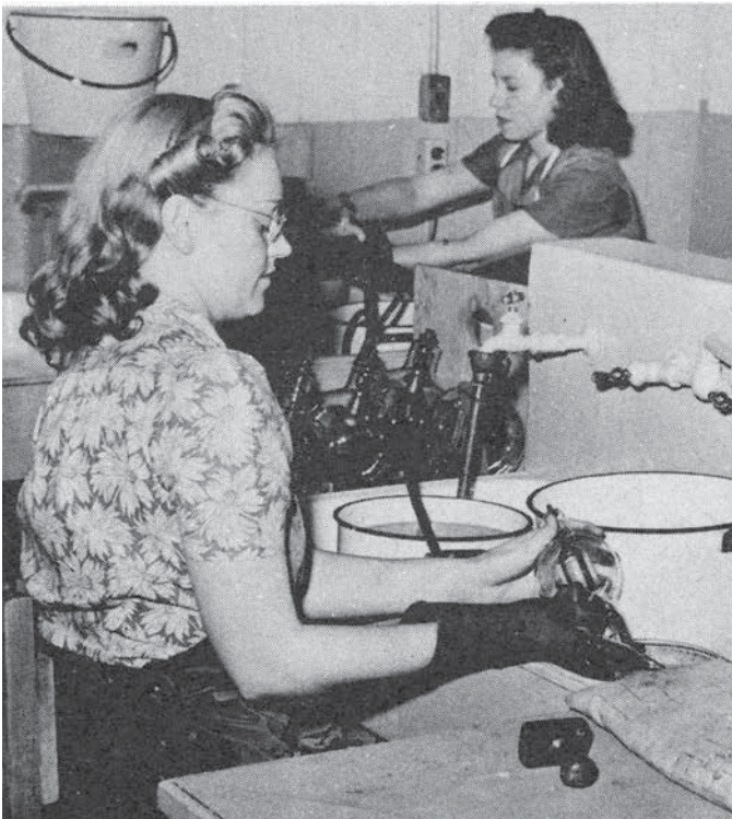
The Chemical Department uses 25 kinds of acid solutions and liquids to clean the tubes. From Eimac News , Tenth Anniversary Edition, September 1944.
