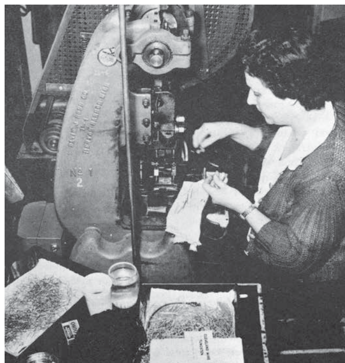
The Punch Press Department forms metal into the shapes needed for the different tube types. From Eimac News , Tenth Anniversary Edition, September 1944.
