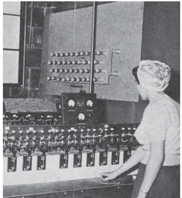
Standards Control samples completed tubes at random to make sure they meet Army-Navy specification. From Eimac News , Tenth Anniversary Edition, September 1944.
