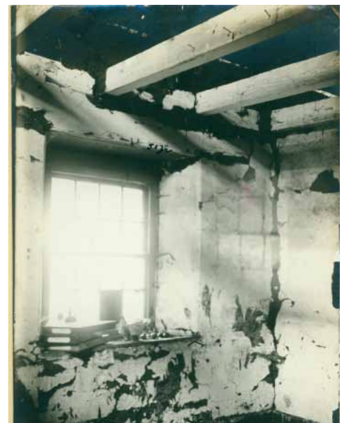
The thickness of the adobe walls can be seen at the windows.
