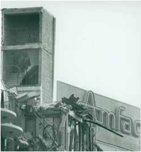
The Amfac Hotel on December 9, 1989. Photograph by Rod Searcey.
