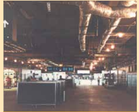
The San Francisco International Airport needed repairs due to water damage from the sprinkler system
