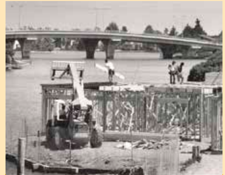
Framing a home in Foster City, 1988.
