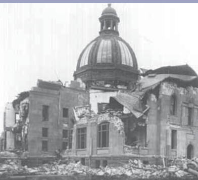
Before the third courthouse could be used, it was destroyed by the 1906 San Francisco Earthquake. The second courthouse (r) was also destroyed.
