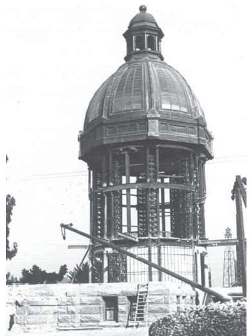
After the earthquake debris had been removed, the dome still stood, c. 1907.
